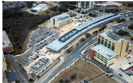
STRF 16 Jan 2011: Note solar panels on roof.
